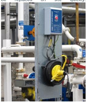
Figure 4: Installed EKX-4 with explosion-proof Cable Reel KA and Grounding Clamp EZI
